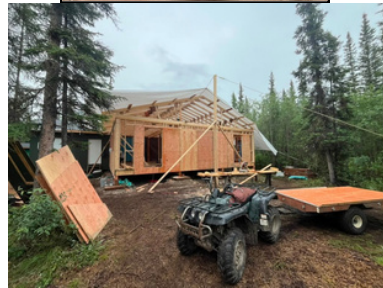
Build trip - adding extension to cabin for the Bible camps
